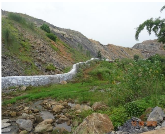
Photo: Photo of retaining wall at the toe of OB dump
